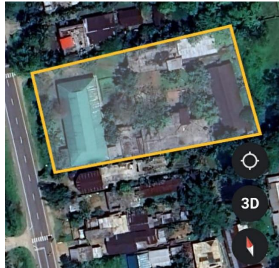
Fig. 2 (b) Hostels and Auditorium
